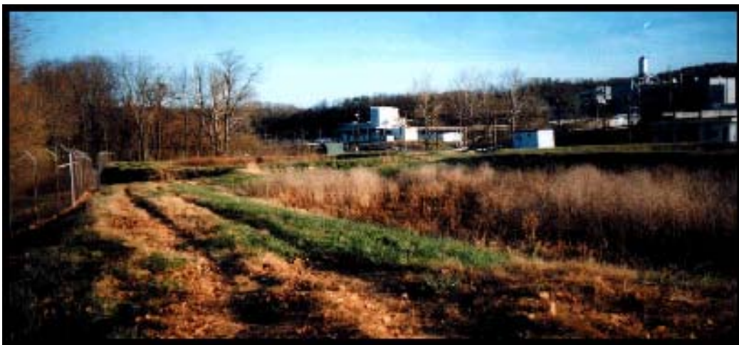
SWMU 36 - CAS04 DRYING BED
