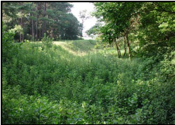
SWMU 38 - CAS04 DRYING BED
